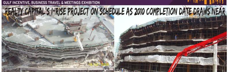
Realty Capital has announced that construction on its centerpiece i-Rise business tower project remains on schedule and will finish on time for the tower's announced mid-2010 completion date. The casting of the tower's 4th podium floor slab is underway and will be completed within a week, while works for the 5th podium level are already in progress. Mechanical, electrical and plumbing installations as well as block-works are also on going at the basement and podium levels.
