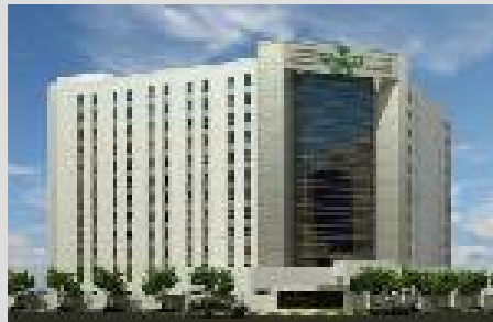
In addition to the 270 king and twin bedded guest rooms and suites, Acacia Hotel also has 103 one-bedroom apartments, each with fully equipped kitchenettes and living-dining rooms. Al Hamra
